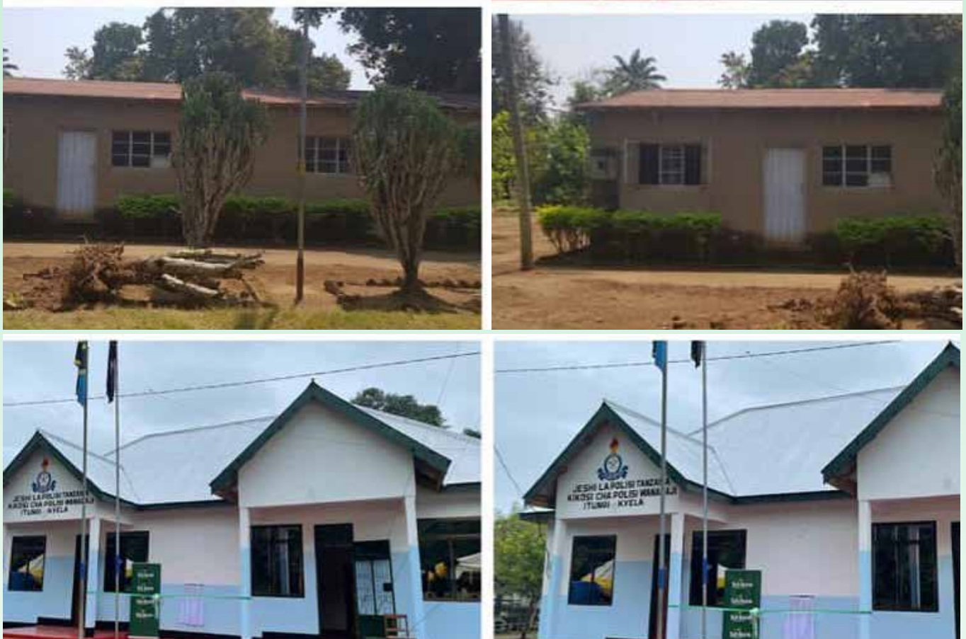
The photos above depict the police station that was renovated by TCB Bank at Kyela, Mbeya Region
