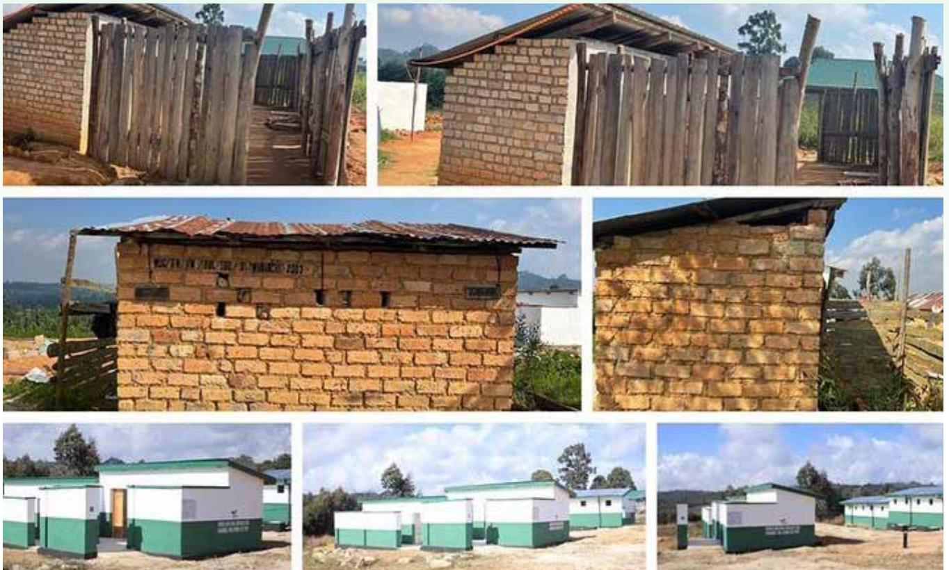
The photos above depict the lavatories built by Tanzania Commercial Bank at Ifwagi Primary School in Mufindi District, Iringa Region
