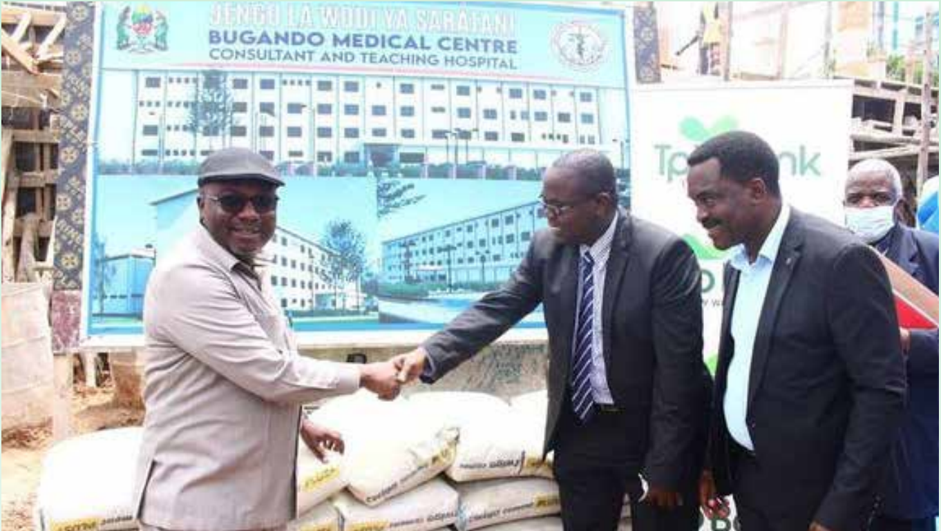
Tanzania Commercial Bank has donated 25 tons of cement bags to Bugando Referral Hospital in Mwanza Region to contribute to the construction of a cancer ward at the hospital. The grant was handed over by the CEO of Bank Mr. Sabasaba Moshingi as detailed in the picture above.
